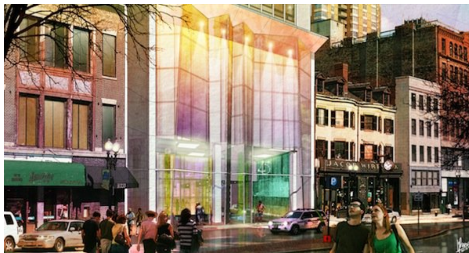
CBT Architect's 45 Stewart Street, the building's podium is cloaked in a five-story glass curtain wall
